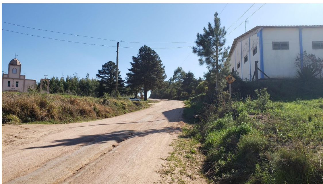
Figura 7 – Rampa superior 7% (PIV-55 – km 14+885)
